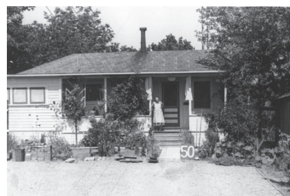
Rear cottage, Parcel 2917
