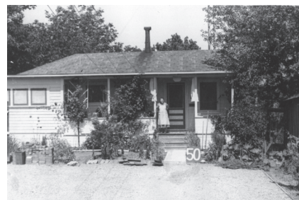
Rear cottage, Parcel 2917
